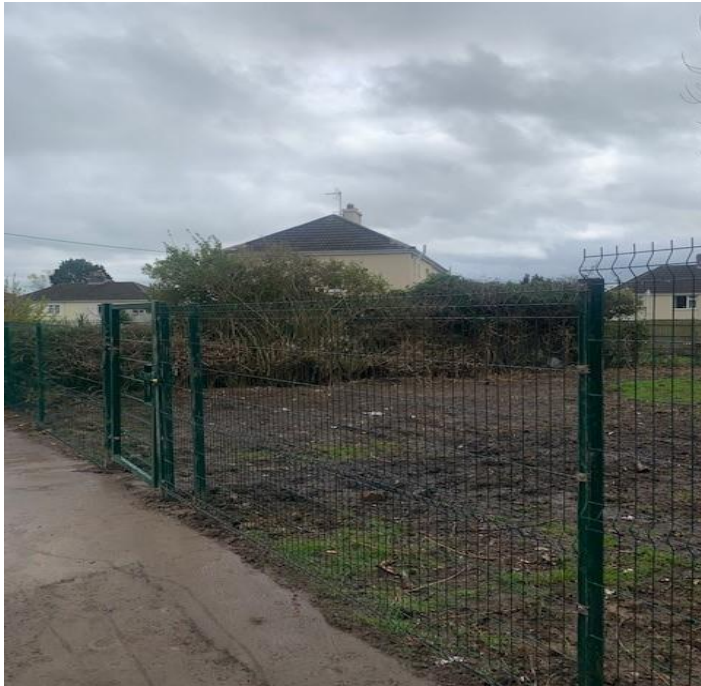
New Fence and Gate installed by SMK Contractors
